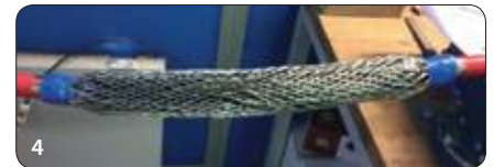
4 The metal shield is rebuilt
