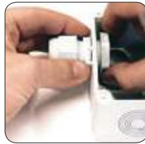
Install the cable glands.
