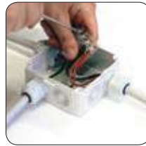
Insert the cables and connect the wires.
