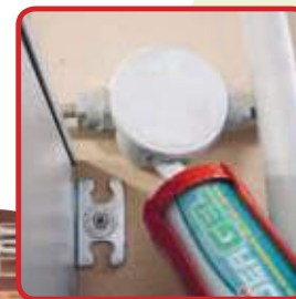
CONNECTIONS IN MOIST ENVIRONMENTS
