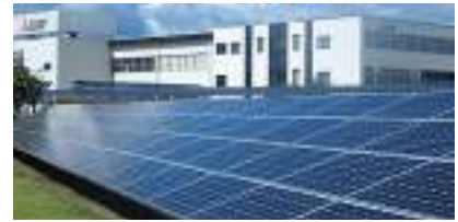
Power Distribution Systems Center (Marugame, Kagawa)
