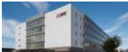
FA Development Center (within Nagoya Works)
